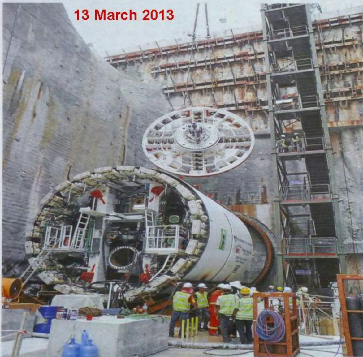
Halfway there: The cutterhead about halfway down the 30m-deep Cochrane shaft.
